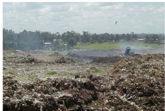
Fig. 1.9: The open waste dump lacks any operational concept and technical provision for protection of public health and the environment (Photo: UV&P, 2004)
