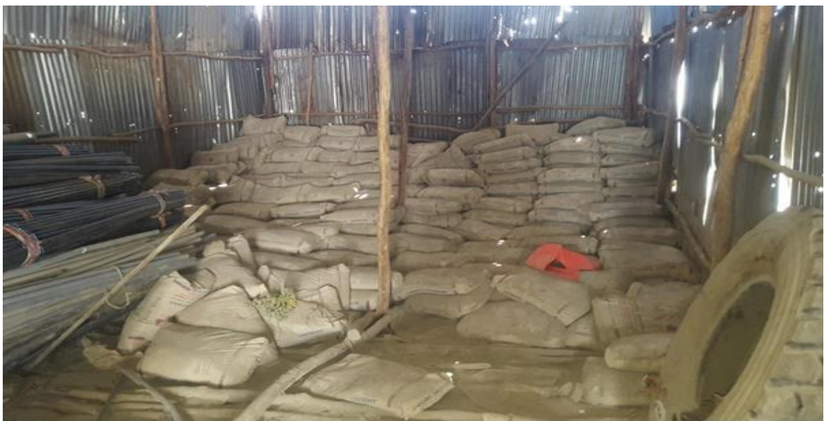
Figure 4.3 improper way of storing cement
