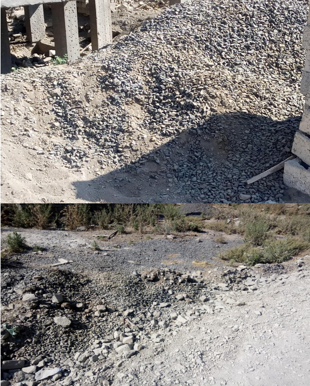
Figure 4.2 wastage of aggregate due to poor storage
